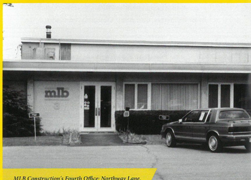
MLB Construction's Fourth Office: Northway Lane.
